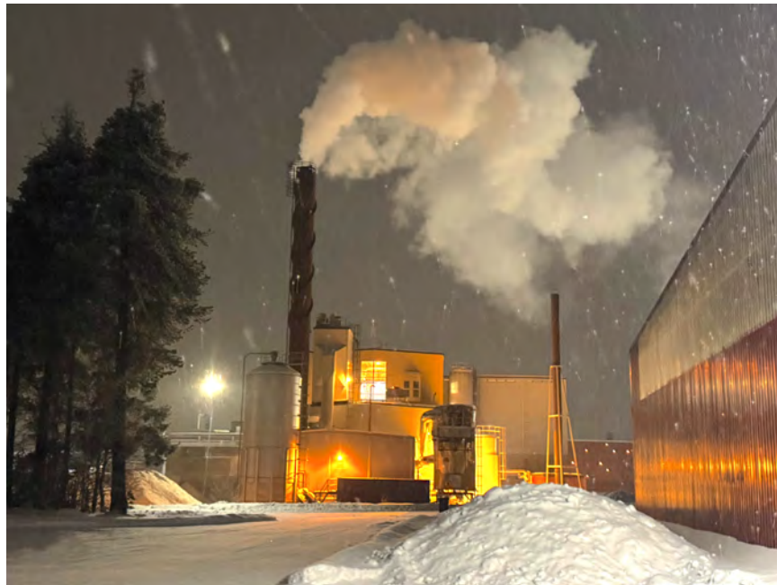
Figure 6: Sawdust from the logging mill in the town of Malå (where historical DUP drill core is archived) is burned to produce hot water for the community
